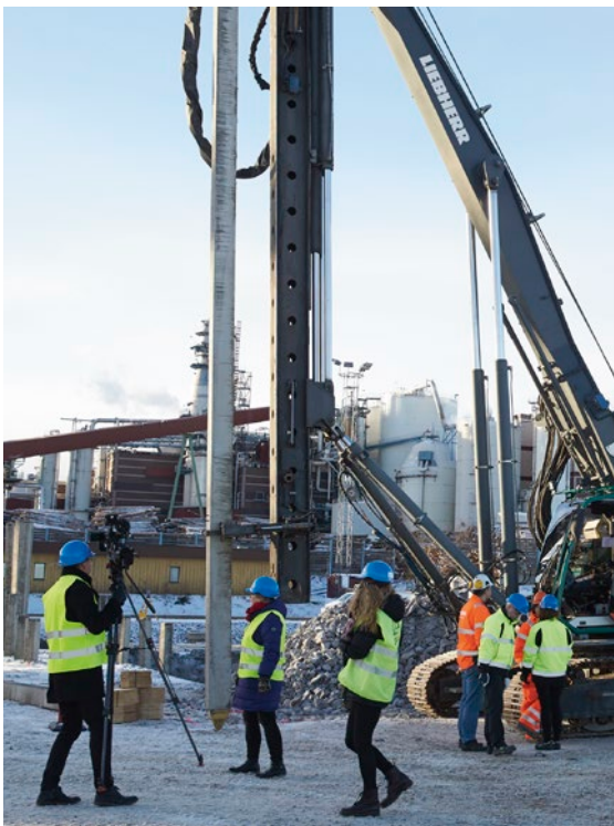
Work on the Östrand project began in February 2016 with a 12 meter concrete pile being driven into the ground.
